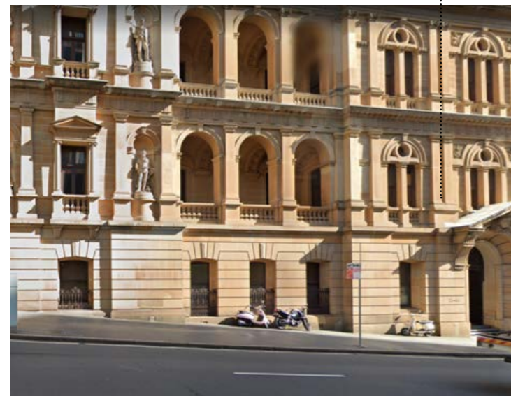
"The Sandstones" buildings (undergoing conversion to high end hotel)
