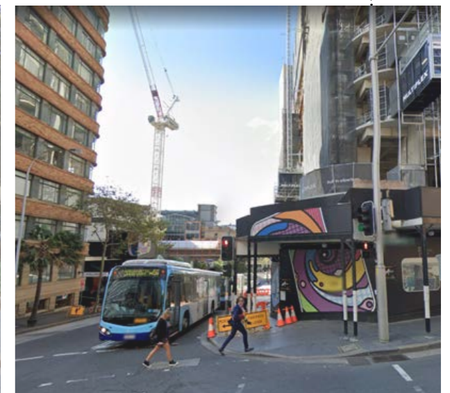
Quay Quarter under construction
